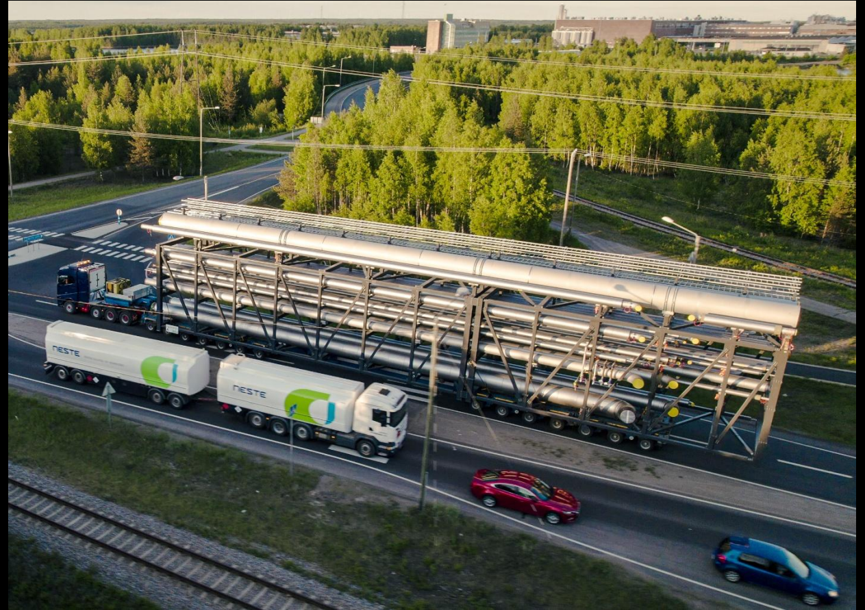
Pipe Bridge Modules
